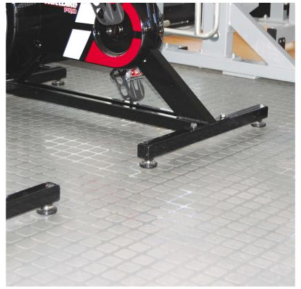
he installation by KBAC lasted two days with the total area serviced amounting to 236m². It entailed the use of 3mm thick Quadra Super Mist 300 x 300 mm tiles. Being PVC and not rubber-based, Transit tiles do not absorb mineral oil-based liquids which together with inherent rubber flooring installation difficulties can cause unsightly 'blistering'. In most instances they can be fitted using a one-way-application, acrylic adhesive, and the entire Transit range is non-directional.
